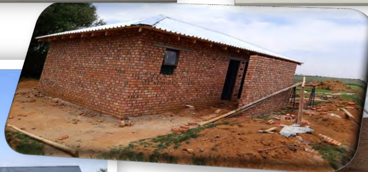
Taung Ablution Facilities renovations
