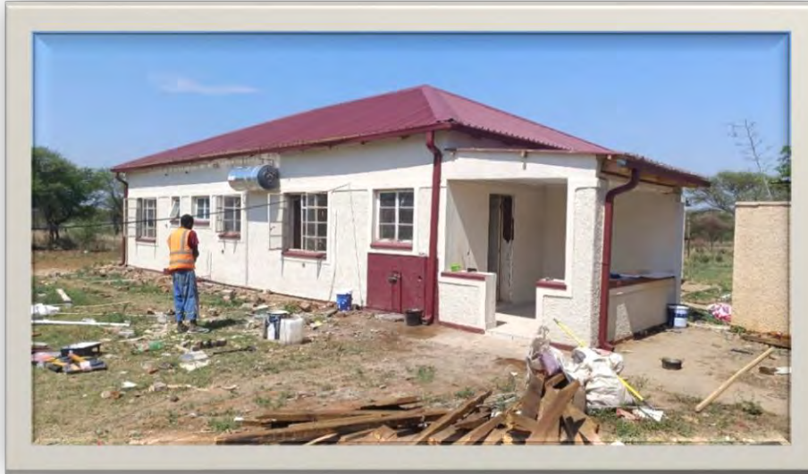
Klipkuil Research Farm single quarters refurbishments
