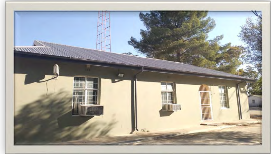
Armoedsvlakte Research Farm renovations
