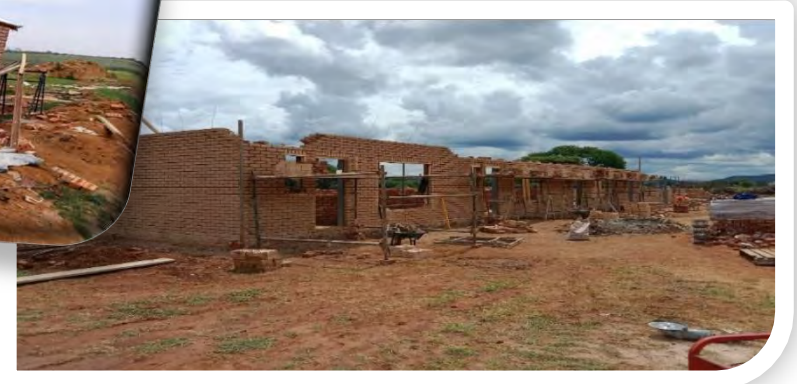
Klipkuil Research Farm renovations
