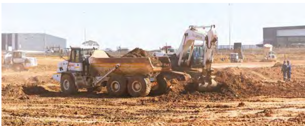
Precinct 2 bulk infrastructure development
