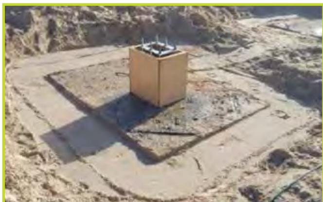
Backfilling around the Foundation Bases. Taken on the 20th of June 2025.
