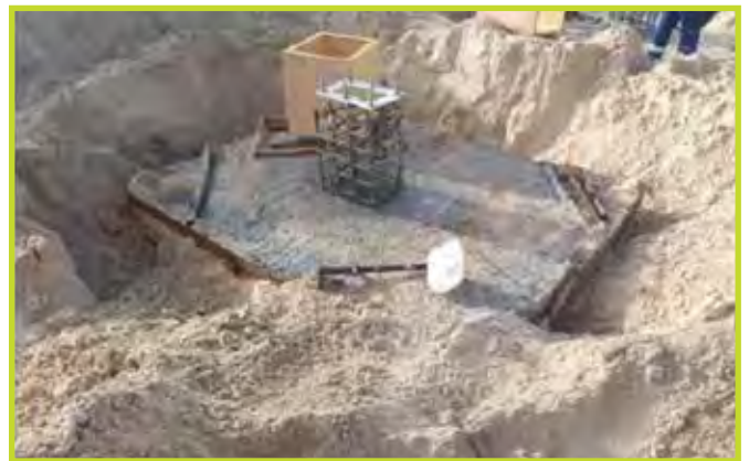
On-going Works: Stripping of Base Formwork and Setting Column Formwork. Taken on the 20th of June 2025.
