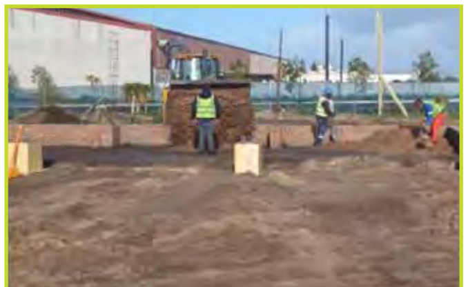
Backfilling on the Office Block's Sub-structure. Taken on the 20th of June 2025.
