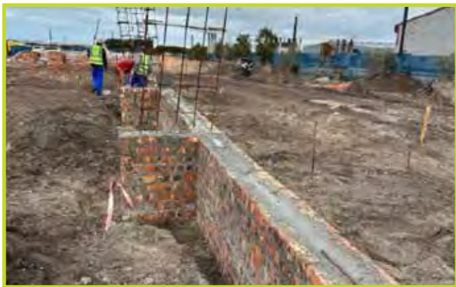
Front portion of the Office Block Foundation Sub-structure completed. Taken on the 19th of June 2025.
