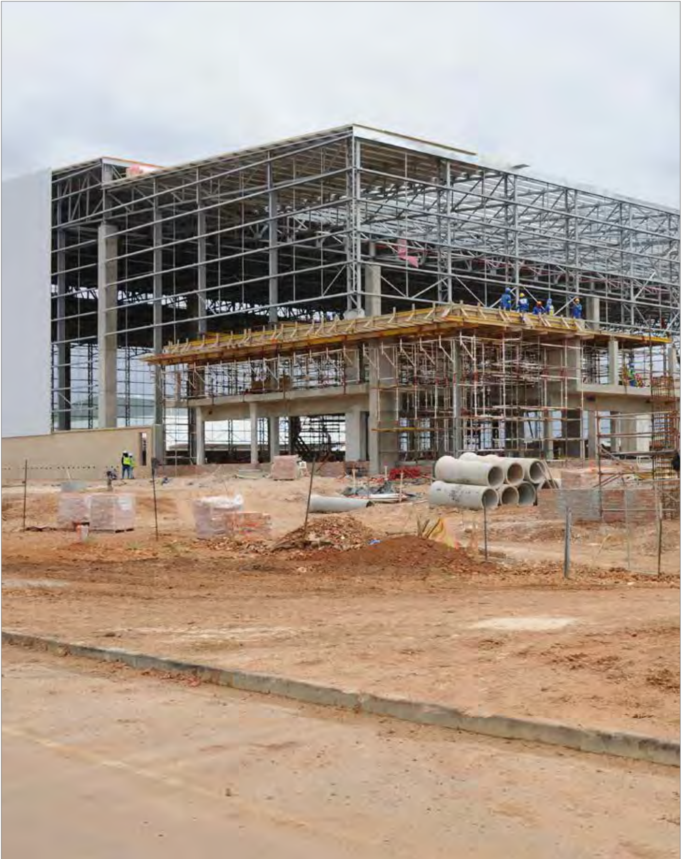
The DHL / Mondelez Facility being constructed in Zone I of the Coega SEZ.
