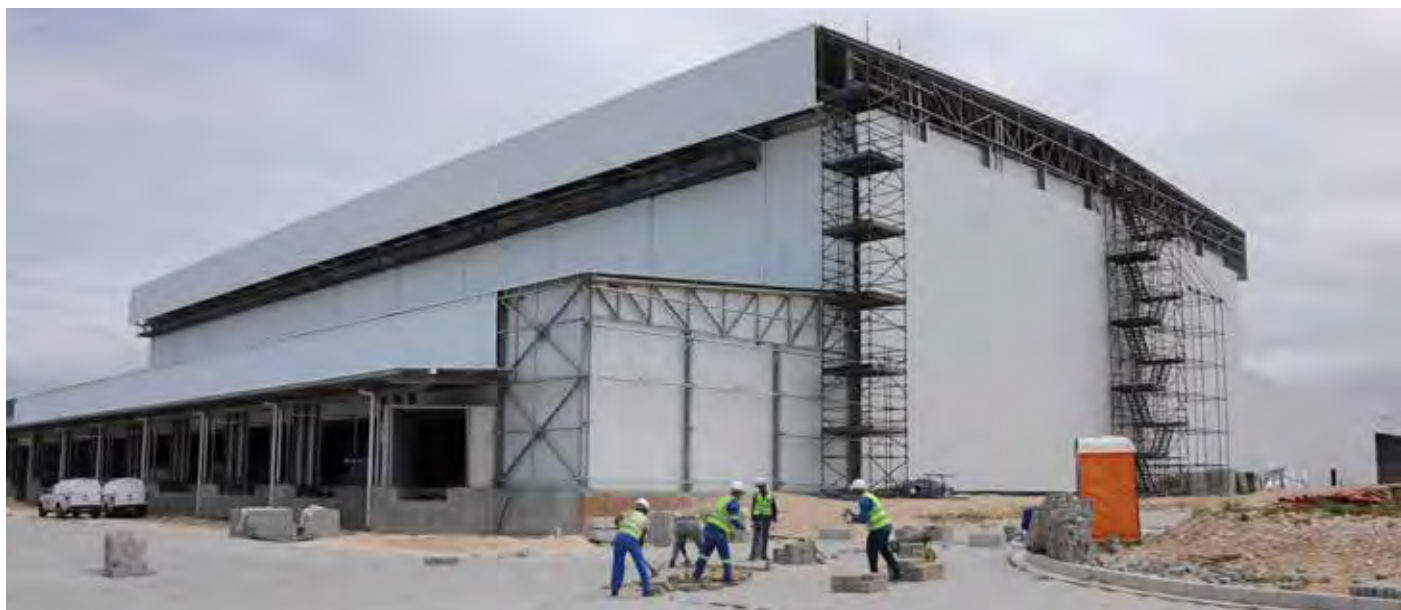
APLI Fruit Terminal construction progress in Zone I.
