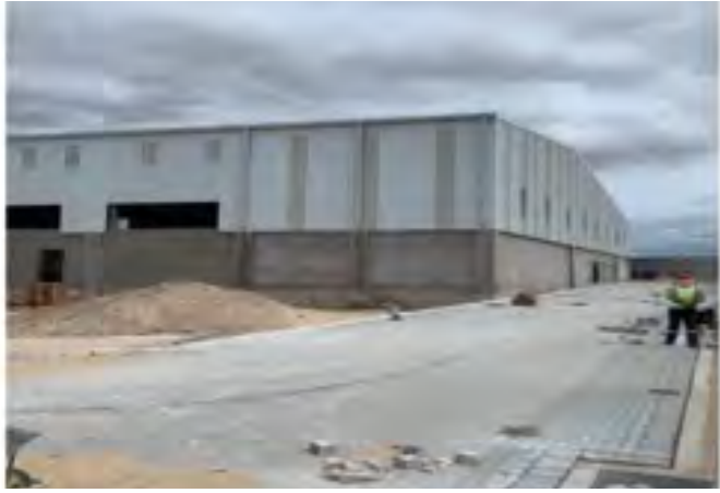
Seraphim Solar Cell Manufacturing Facility in Zone 3, Coega SEZ.
