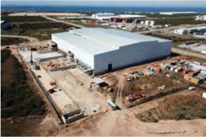
DHL / Mondelez Facility in Zone 1, Coega SEZ.
