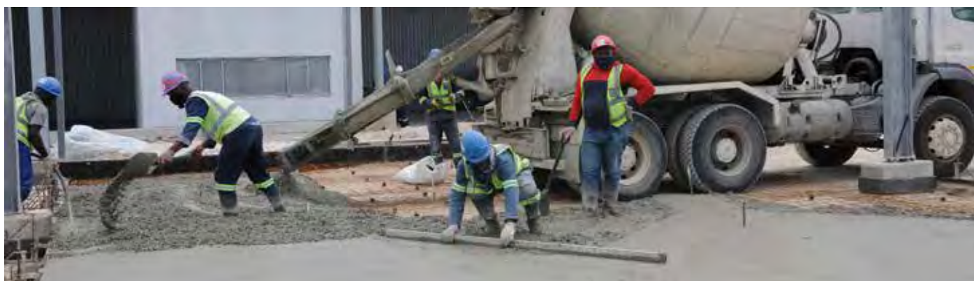
APLI COLD STORAGE: SMMEs working to complete the Fruit Terminal.
