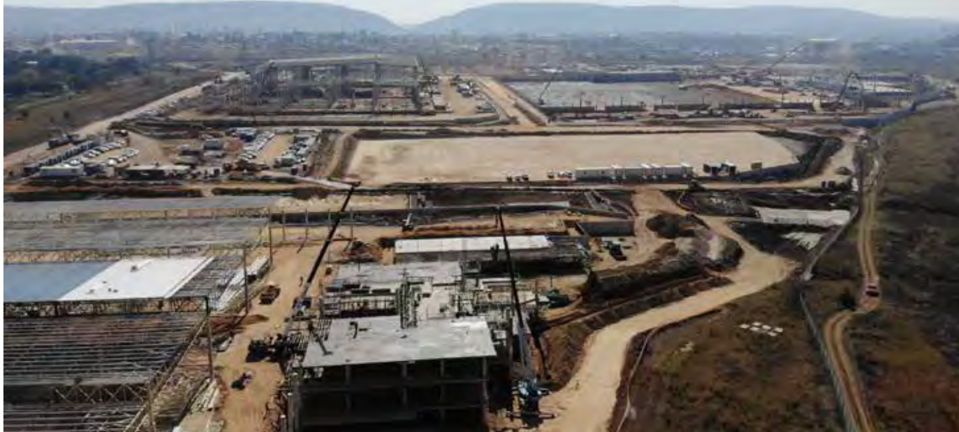
Aerial view of the Tshwane Automotive SEZ, Phase I, construction progress to date.
