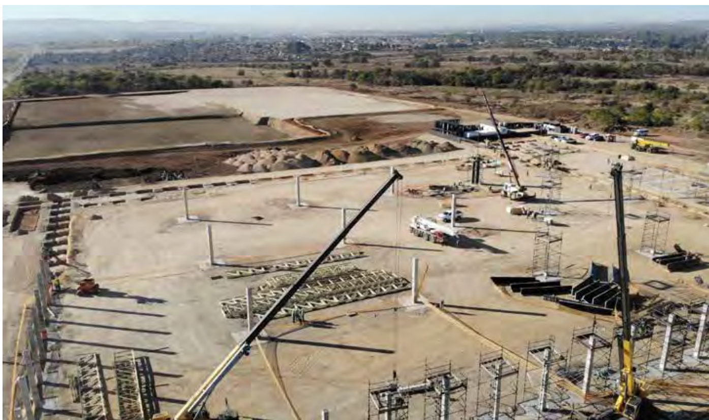
Aerial view of the Tshwane Automotive SEZ, Phase IA, construction progress.
