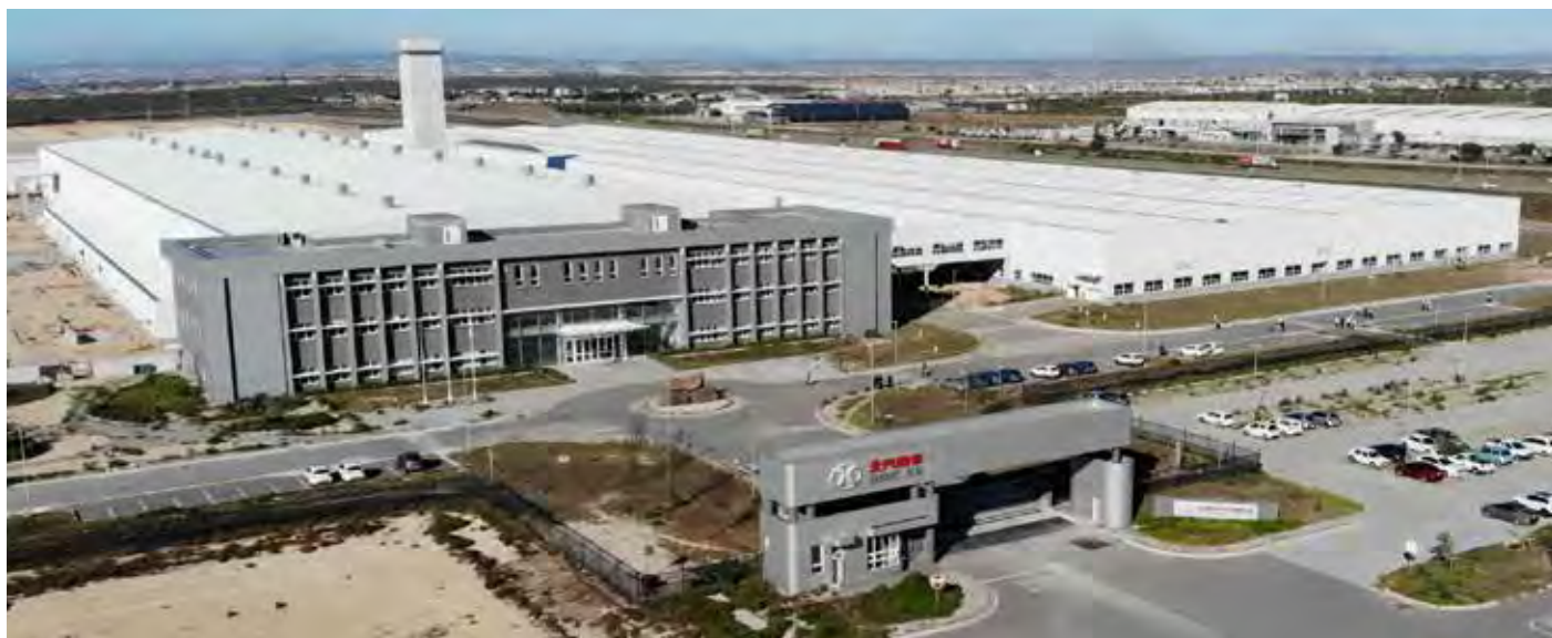
Aerial view of BAIC SA construction progress in Zone I.
