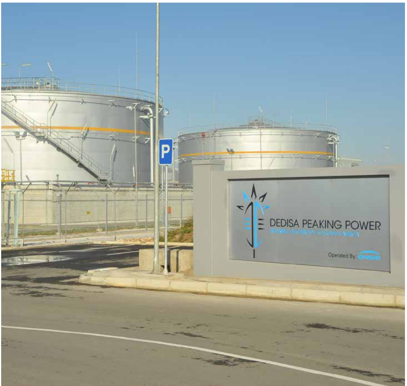
DEDISA PEAKING POWER PLANT: Located in Zone 13 of the Coega SEZ.
