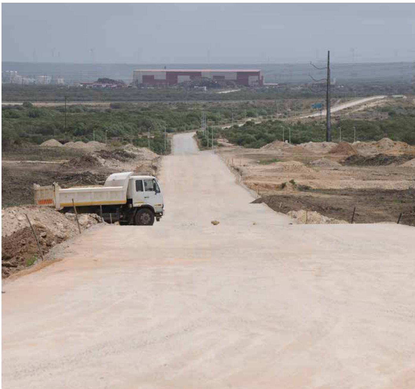
New Aquaculture Development Zone - Infrastructure Development in Zone 10, Coega SEZ.
