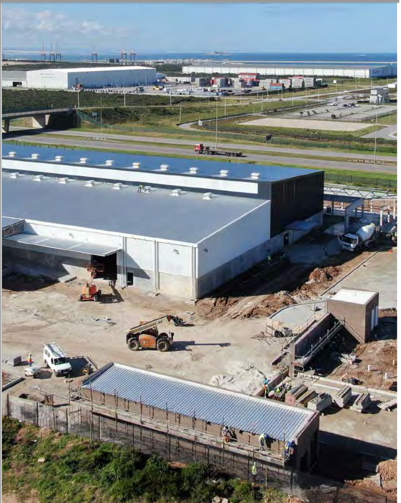
Progress being made on the Weidplas Automotive Plastic Component Manufacturing Plant in Zone 2 of the Coega SEZ.
