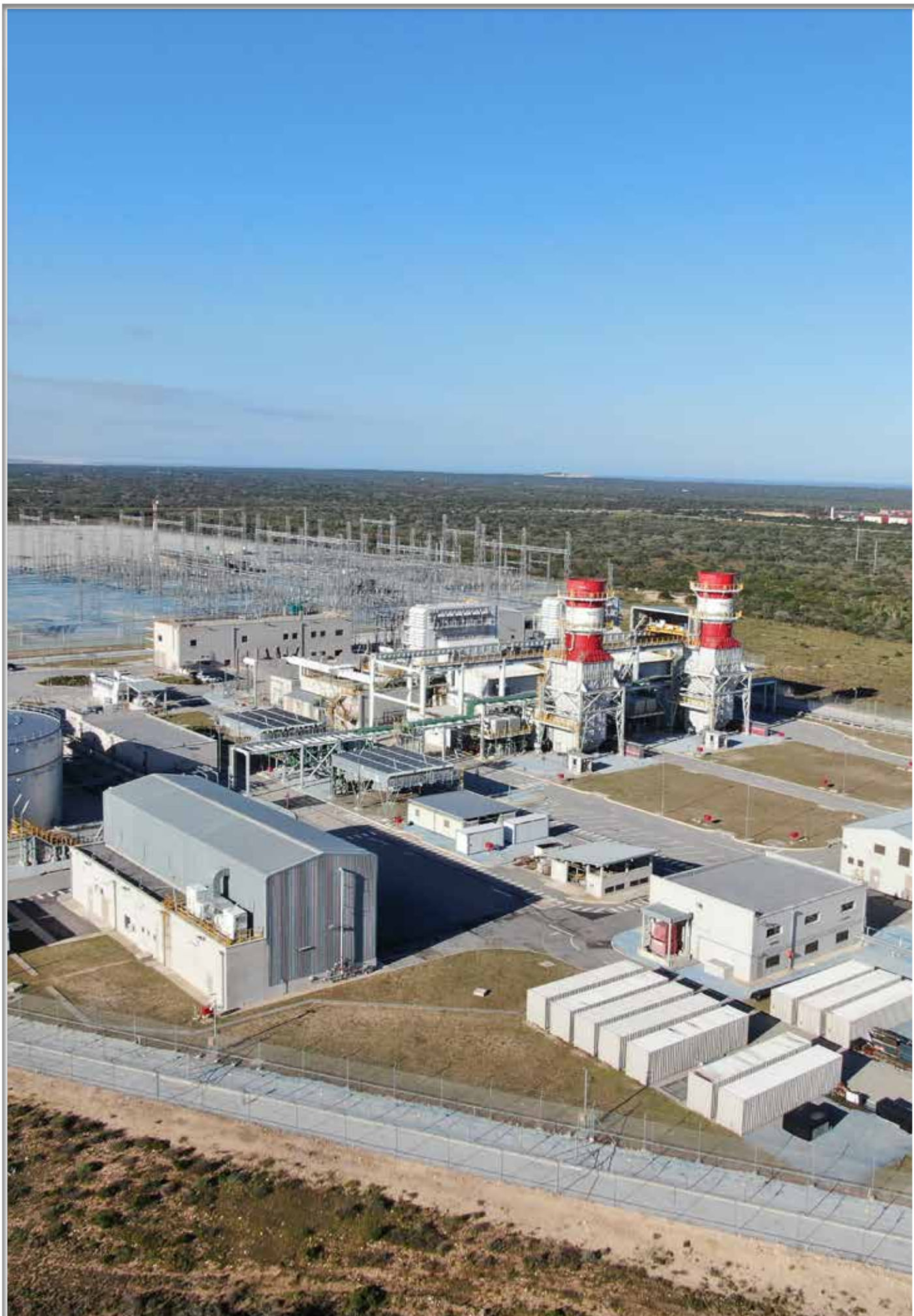
The Dedisa Peaking Power Plant, in Zone I3 of the Coega SEZ.
