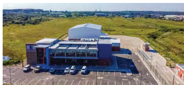
Photo: Nyanza Product Testing and Development Centre (PTDC)
