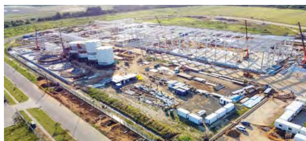
Photo: Wilmar Processing SA Construction Site
