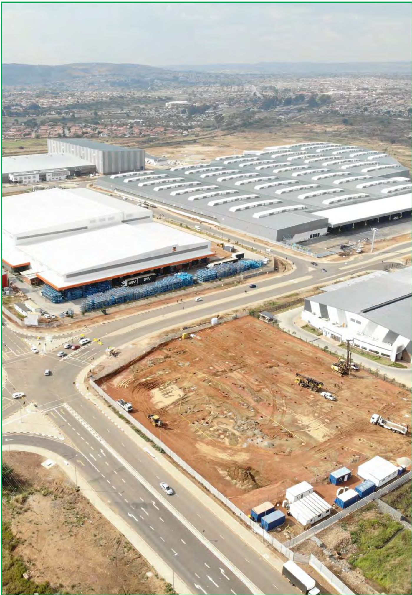
Tshwane Automotive SEZ construction site.
