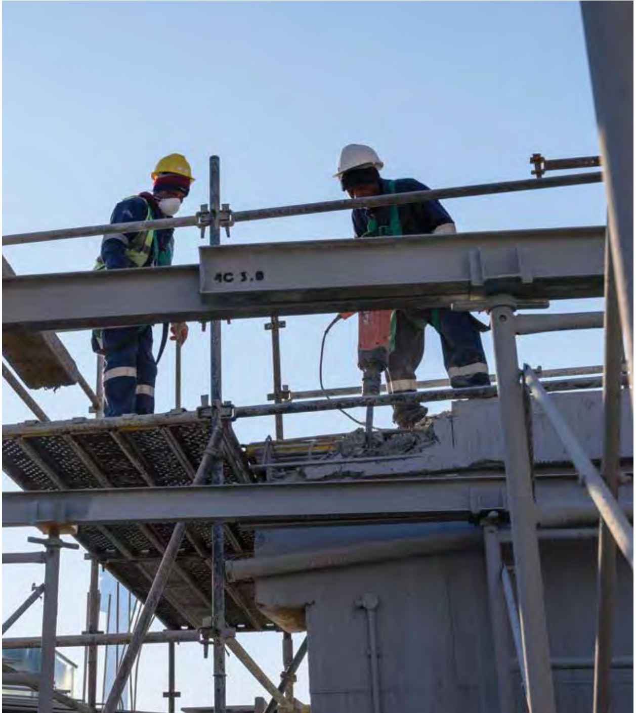
Construction at ConHill Visitors Centre
