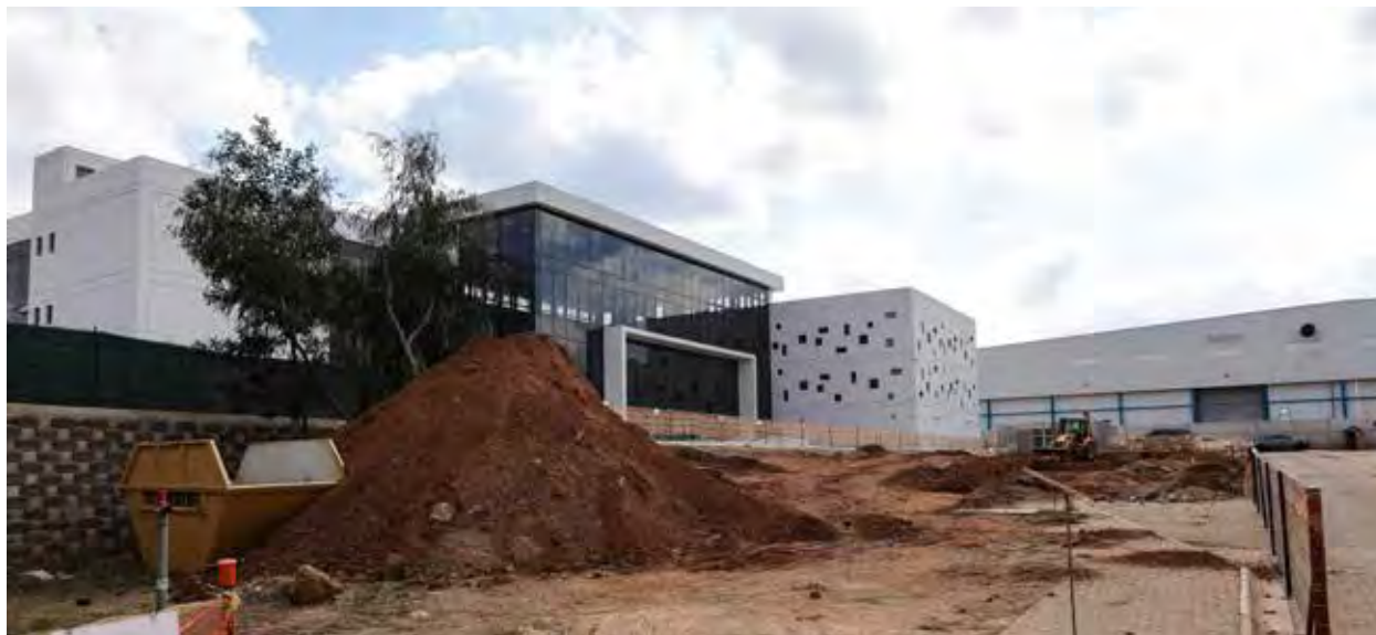
Construction works underway at the OR Tambo SEZ
