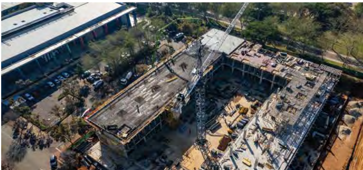
TIH BioPark Phase 3 construction in progress
