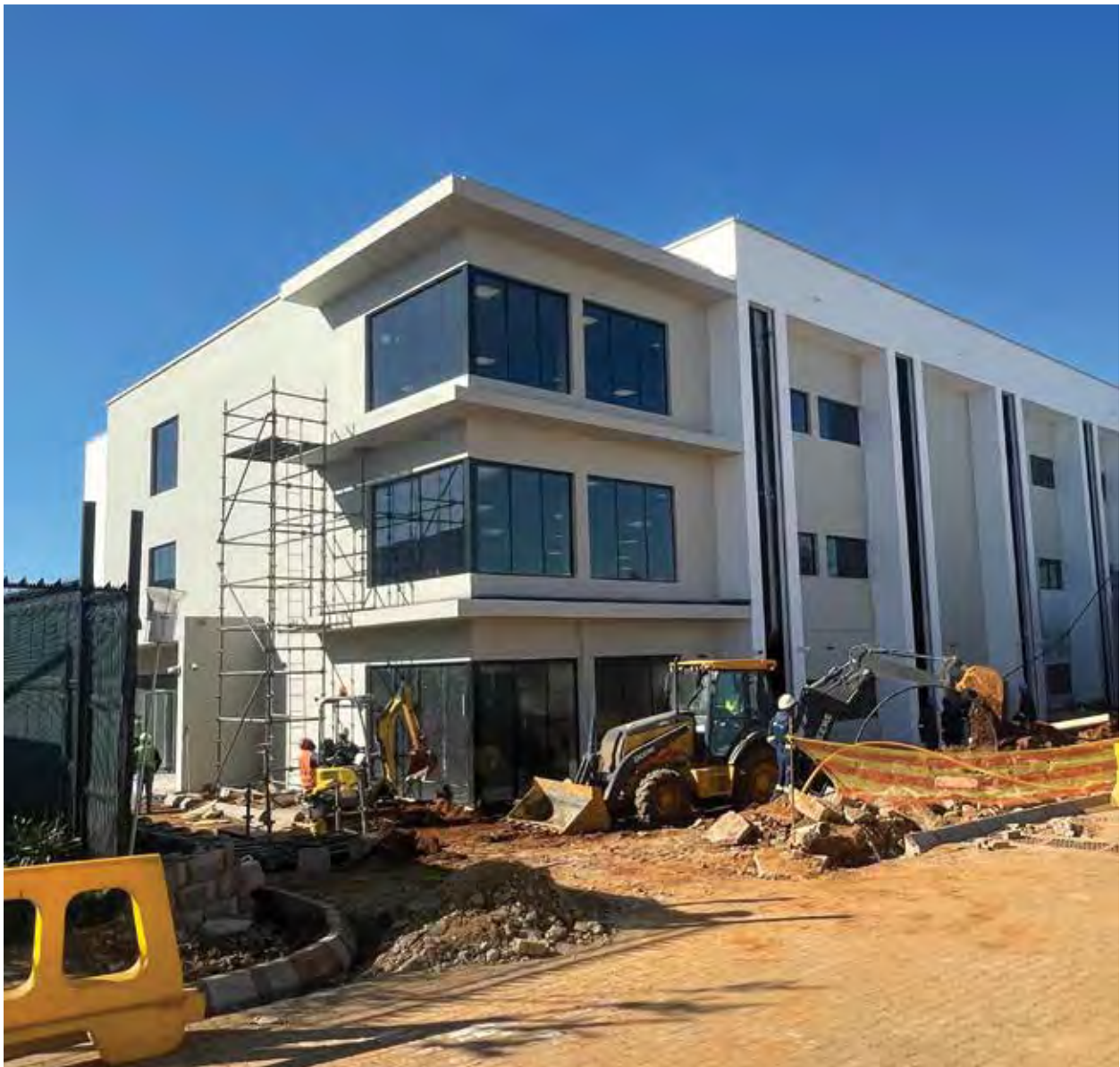
Construction of the Jewellery manufacturing Precinct
