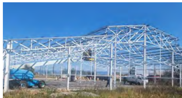
Rebuild at Lot 50 at Madadeni Industrial Estate
