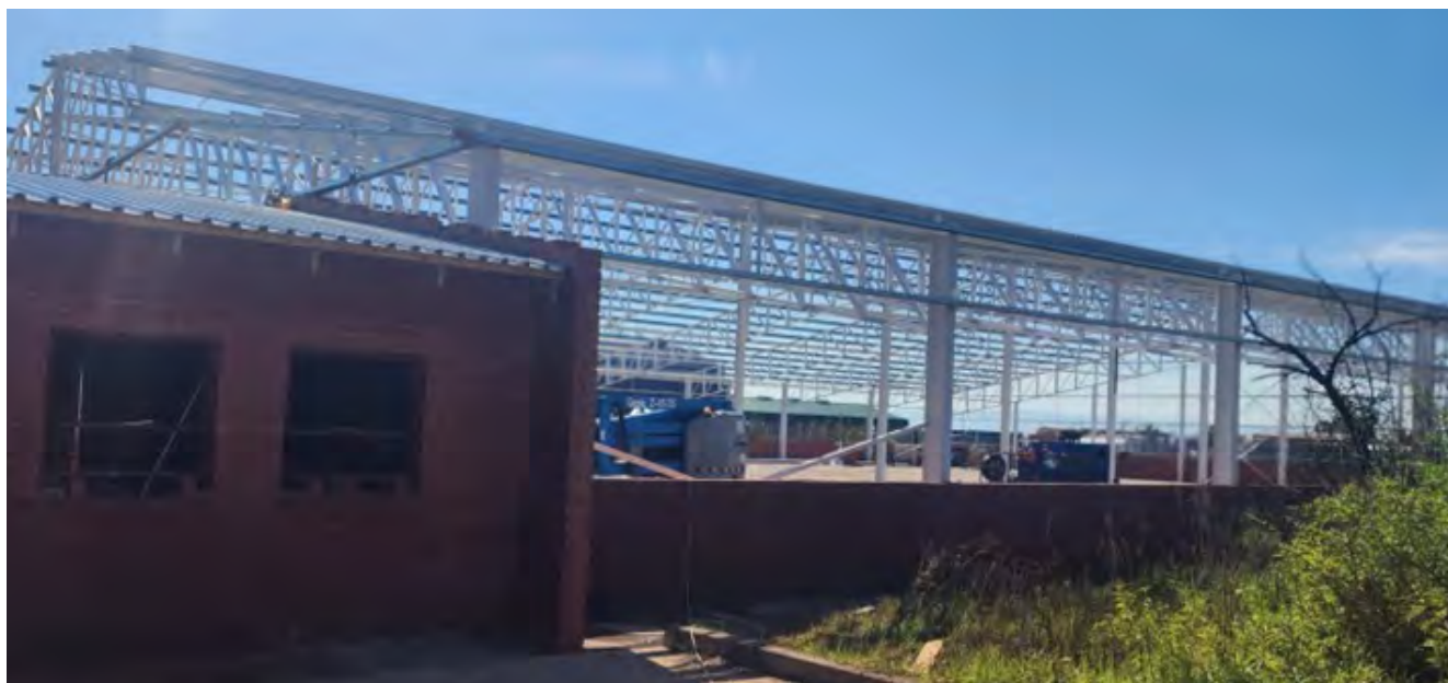
Rebuild at Lot 50 at Madadeni Industrial Estate
