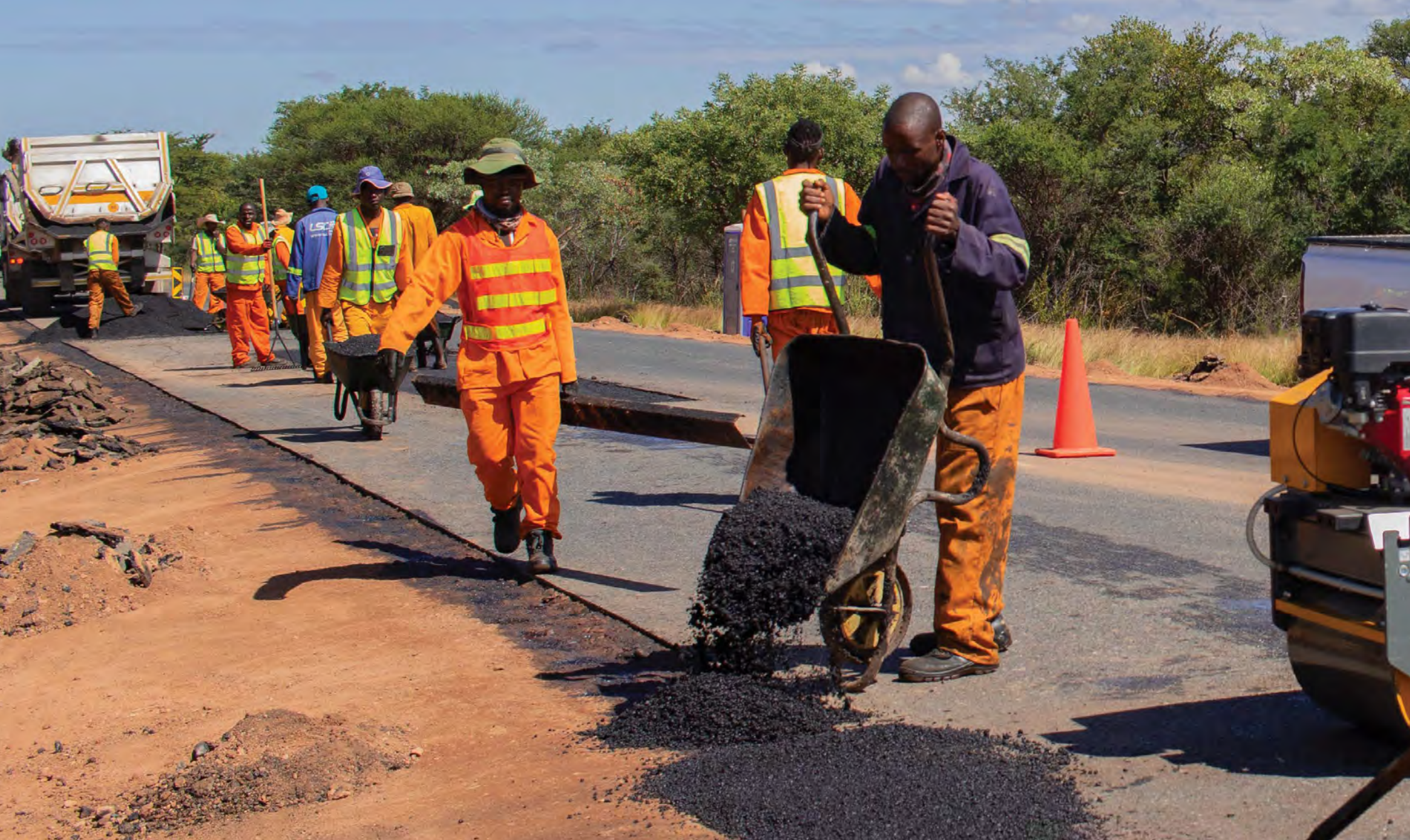
The rehabilitation of road P18/2 (R519) from Zebediela towards Bergenek in the Capricorn District during the 2022/23 financial year has led to the creation of numerous job opportunities for local residents and empowered small local businesses in the area.
