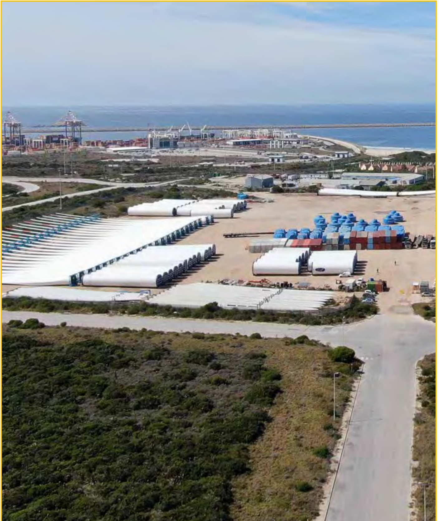
Supporting the Just Energy Transition, Coega has a dedicated Laydown Area for imported renewable energy components in Zone 1 of the Coega Special Economic Zone, next to Ngqura Port.
