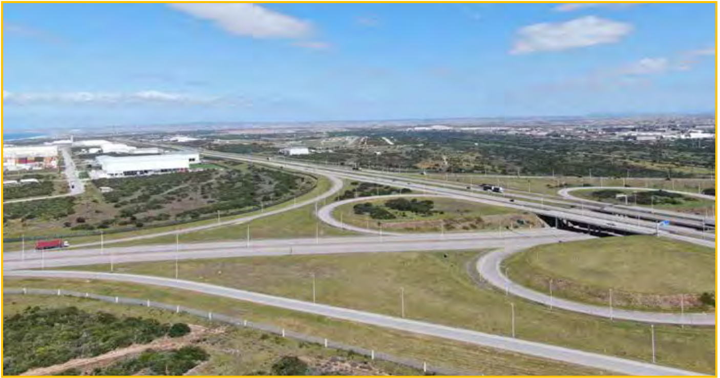
The National Road N2 intersection connecting Neptune Road of the Coega Special Economic Zone, Gqeberha with the rest of the Eastern Cape, South Africa and African continent.
