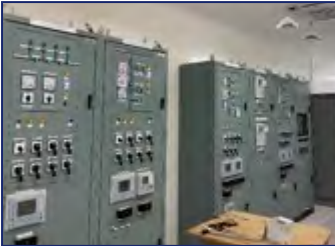
Completion of BAIC Zone 2 HV Electric Upgrades
