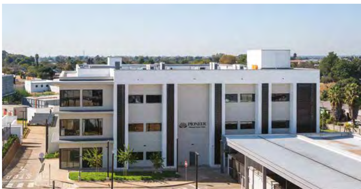
Pioneer Diamond Tender House located at the Jewellery Manufacturing Precinct (JMP) within the OR Tambo SEZ
