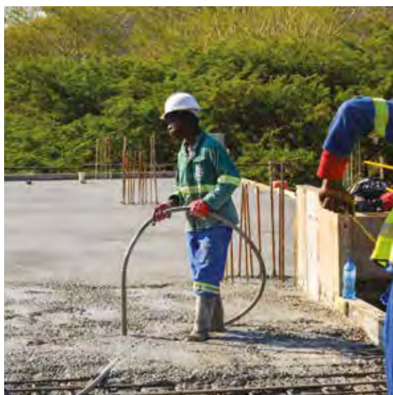
Construction workers at the BioPark
