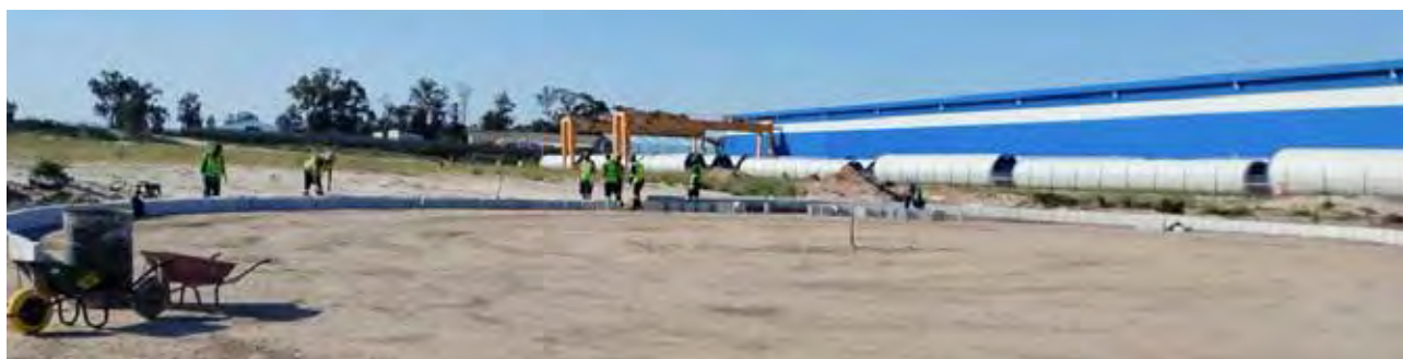
First female SMME onsite: construction of road kerbing and sidewalk paving.
