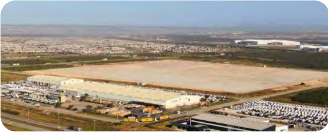
Stellantis Automotive Manufacturing Plant (Zone 2)
